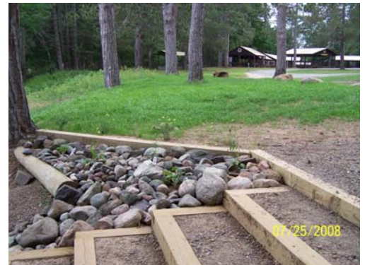
RIGHT: At the top of the steps rocks and timbers along with newly planted grass and flowers will help keep the hillside from eroding away.
