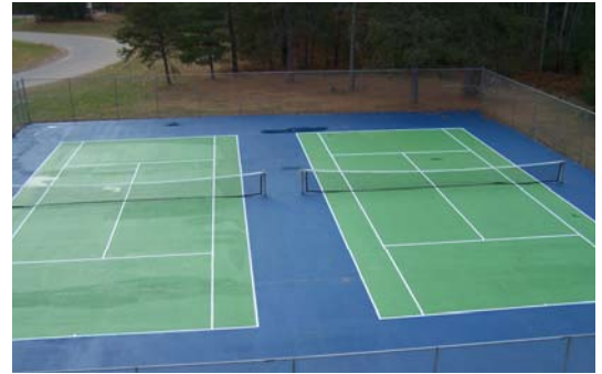
Runkle Lake Park Tennis Courts
